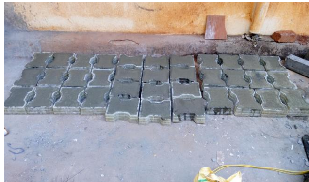
Figure 1: Casting of Paver Block
